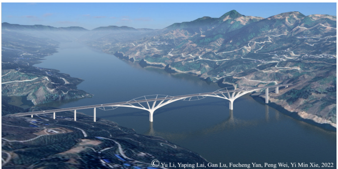
A recent bridge design using topology optimization (by Prof. Xie's team in collaboration with T.Y. Lin International)
